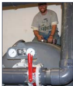
Replacing the sand filter.
